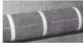
1 FOAMGLAS® Insulation installed with chalk line at three o'clock position.
