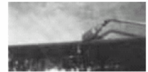
8 Burn off polyester film for distance of 2" on each side of PITTWRAP® jacketing.
